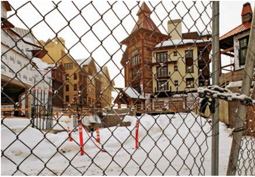
Construction stopped at this Tamarack 'village' when the resort was handed to a receiver.
